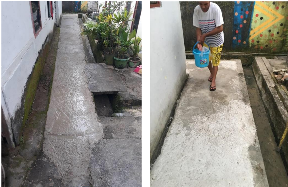
Gambar 3. Proses Perawatan/curing Beton Pasca Pekerjaan
