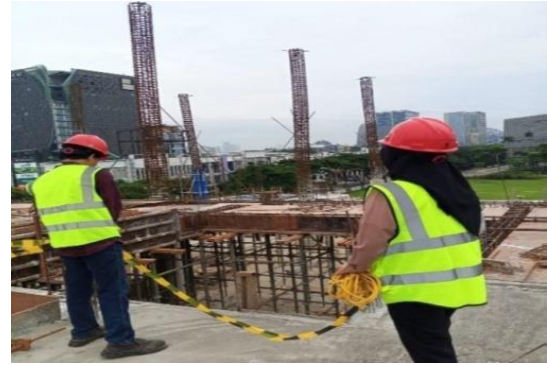
Gambar 4. Pemasangan safety line
